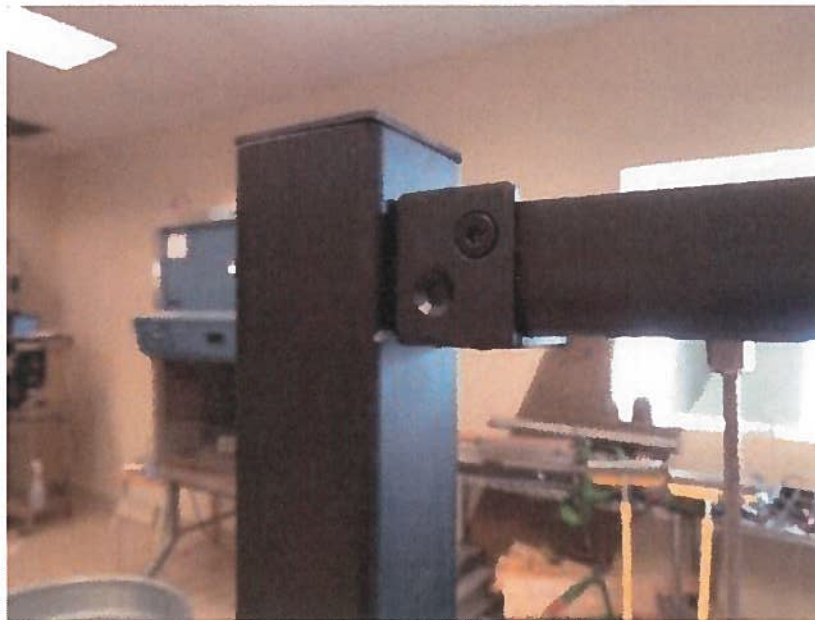
Photo No. 10 Top Rail Universal Bracket to Rail Connections
