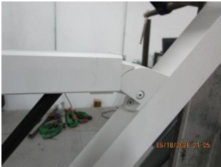
Photo No. 10 Stair Rail Bracket
