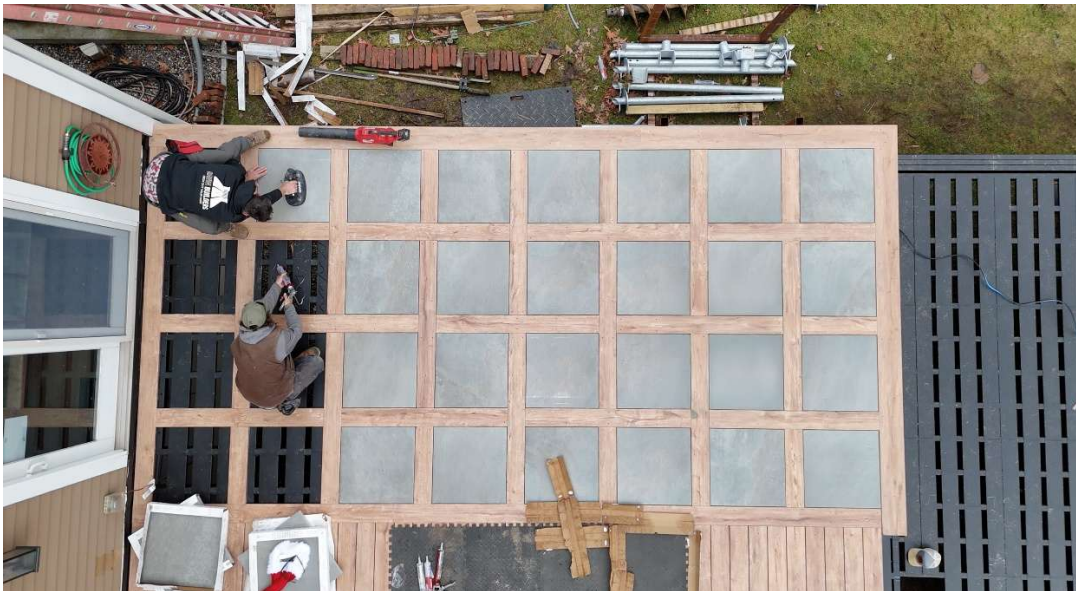
Fig 1: Steel deck frame with outdoor tiles positioned on top.
