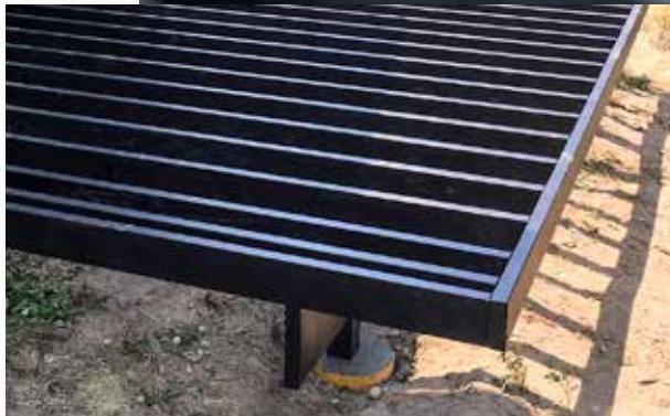
16 Gauge 51mm x 152mm Joist (G60 Galvanised & Black Sand Powder Coated)
