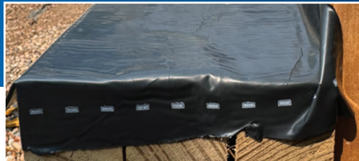
Figure 11: Butyl Tape on the beam before the joists are added.
