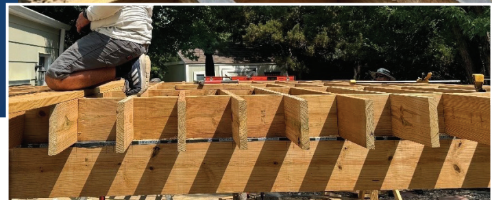
Figure 12: Builder installing the joist tape. Using a board to protect their knees and to make installing the tape easier.
