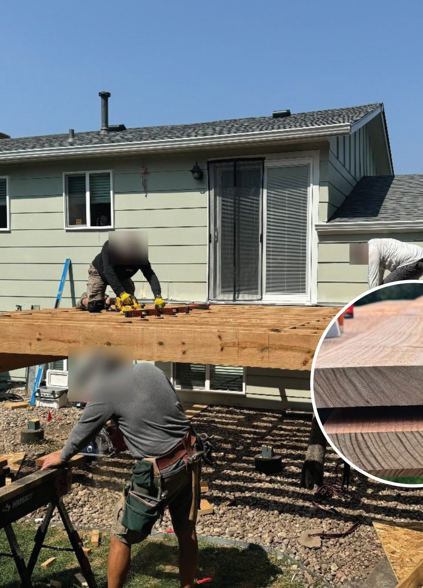
Figure 9: Builders planing each joist to even out the surface.
