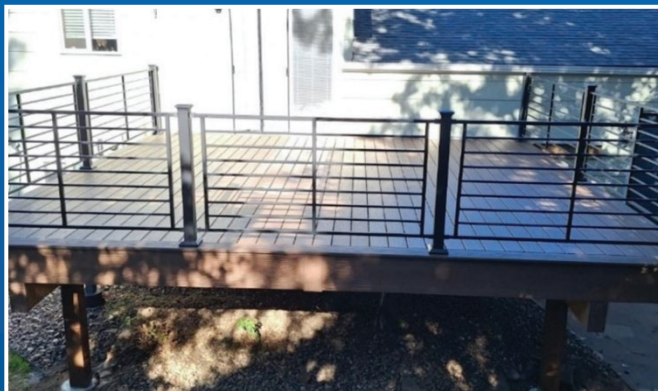
Figure 1: Completed wood build using Kiln Dried PT, Fortress Axis Railing and MoistureShield Vision Decking.
