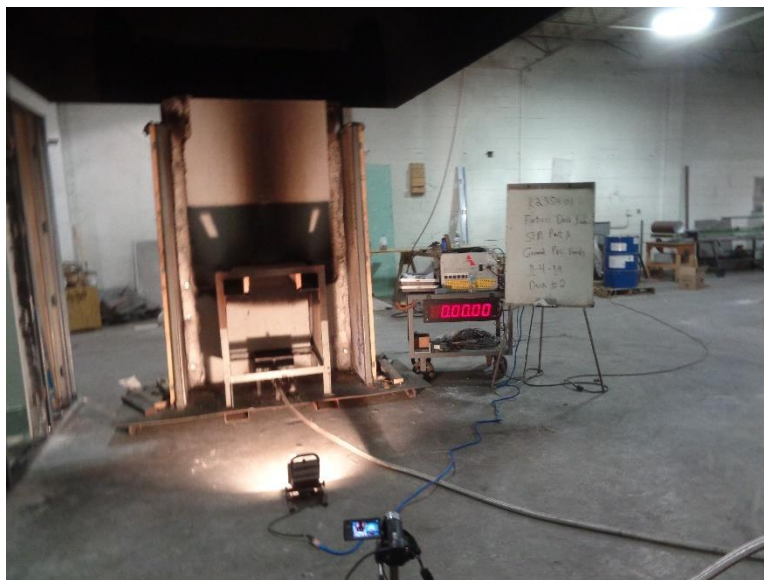
Photo No. 4 Test Assembly (Pre-test)
