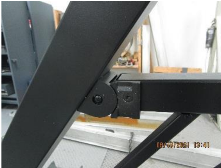
Photo No. 7 Cast Aluminum Bracket for Stair Top Rail
