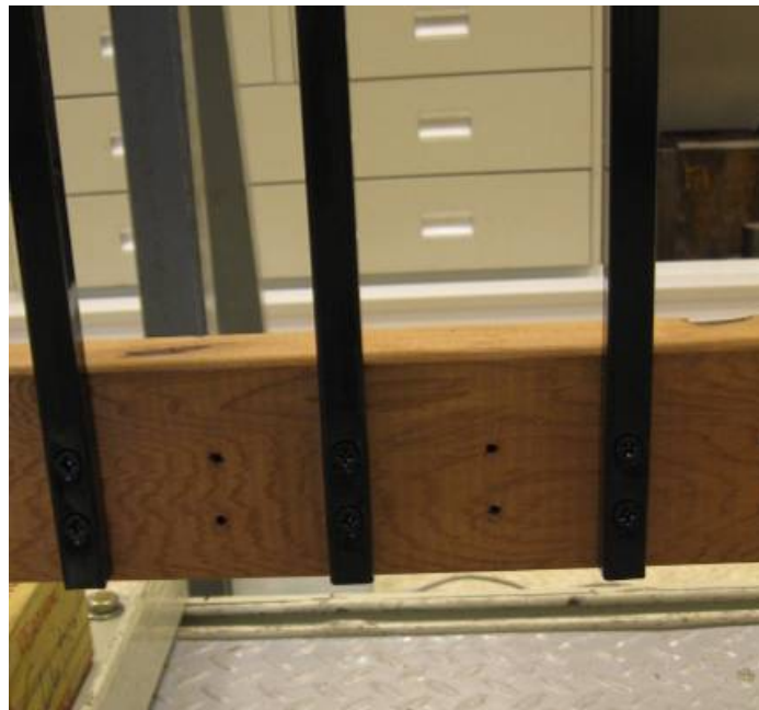
Photo No. 6 Vintage Series Square Baluster Installation (4 in On-Center Spacing)
