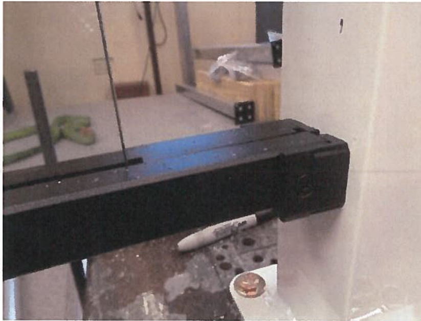
Photo No. 7 Rail Collar Bracket and Post Mount Connection
